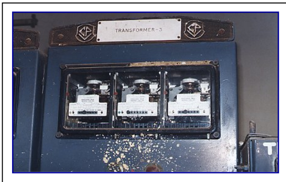
Fig. 1 CDG31 Relay in Service
